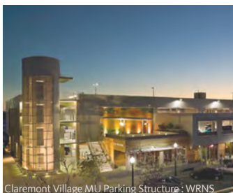
Claremont Village MU Parking Structure : WRNS
