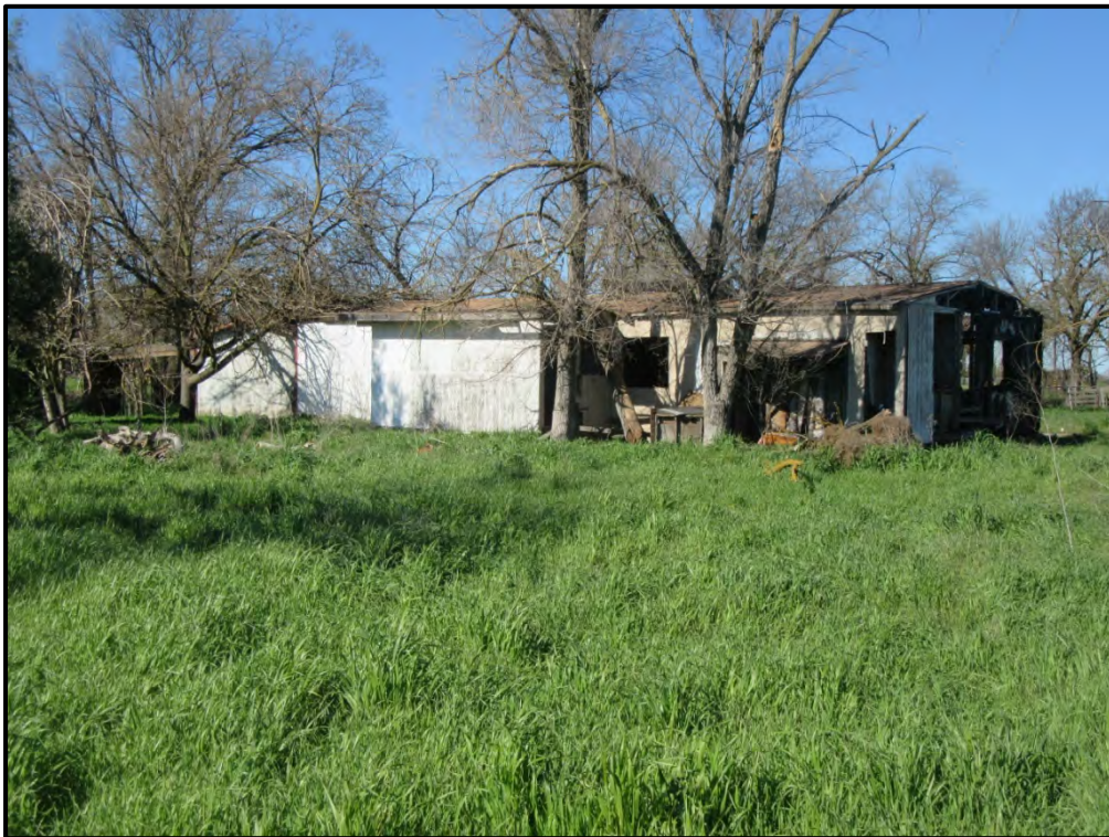
Abandoned residence in the northeast corner of the 20+/- acre parcel, looking northeast; 02/18/19. There are a few large trees and smaller dwellings in this area.
