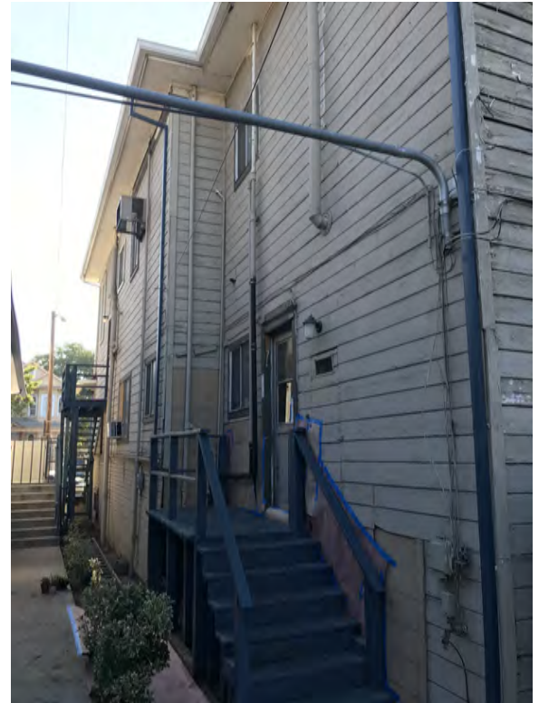
Concerns include wooden first floor exterior stairs, additional exposed plumbing Front, second story stairs are wood
