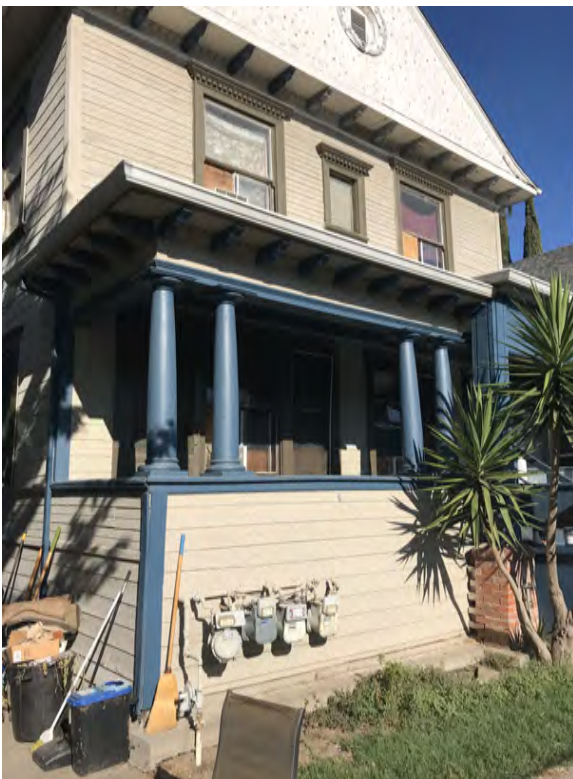
Concerns include front porch foundation settling and wood single pane windows
