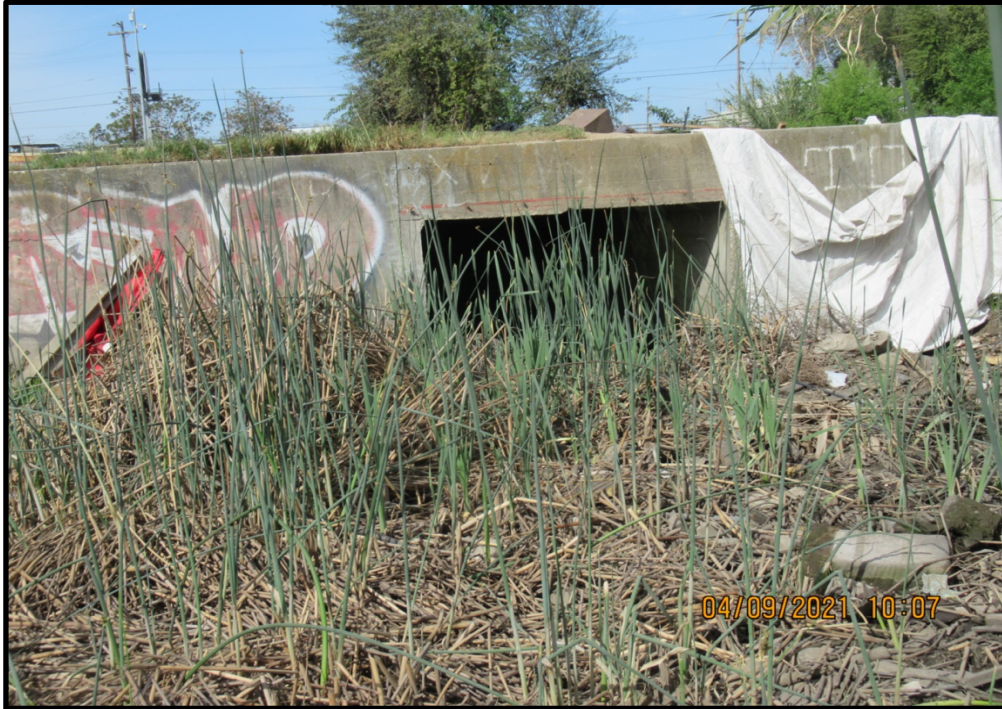
Patch of dense tules at the upstream end of a large box culvert within Mormon Slough; 04/09/21. This is the inlet to a long underground culvert system that conveys flows to the west.
