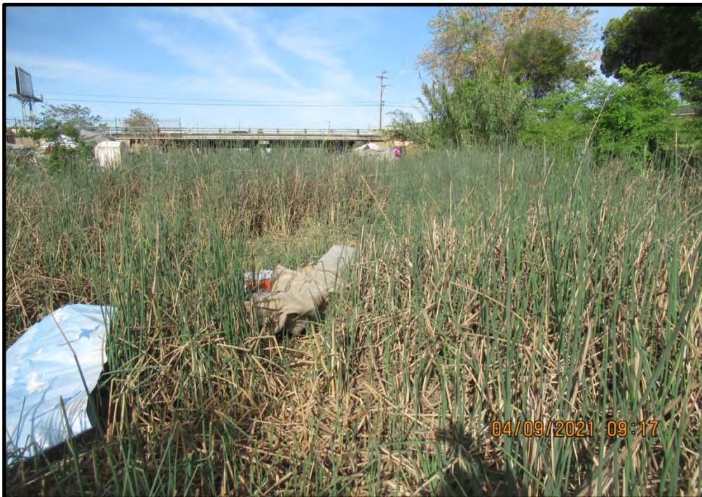
Tule patch downstream of the box culvert inlet, looking west; 04/09/21.
