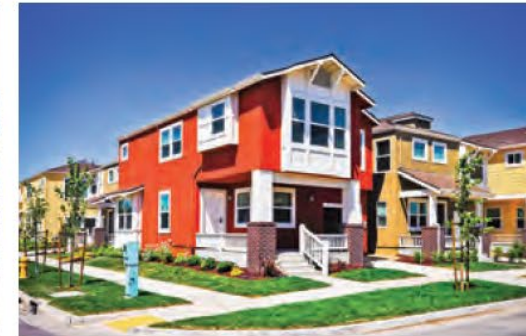
Newly built affordable housing project with duplexes.
