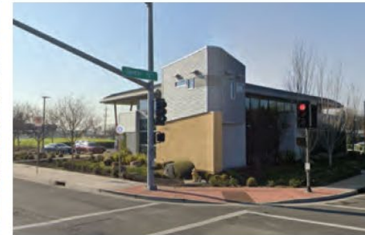
The Financial Center Credit Union at 10th and South Airport Way.
