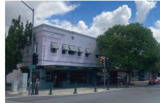
Typical commercial development on Miracle Mile is comprised of one to two stories buildings
