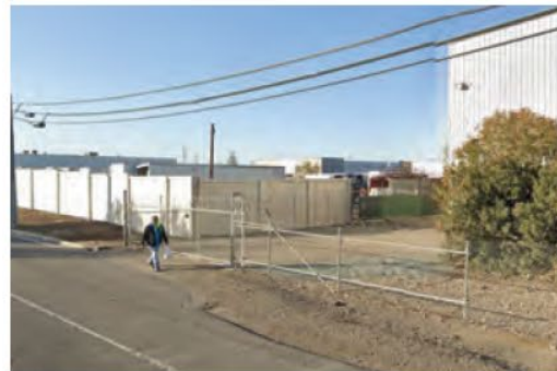
Some older industrial development on South Airport Way does not face the street, and sidewalks are missing.
