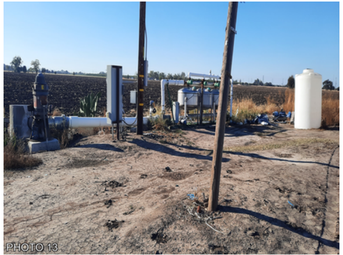
IRRIGATION WELL AND UNKNOWN TANK
