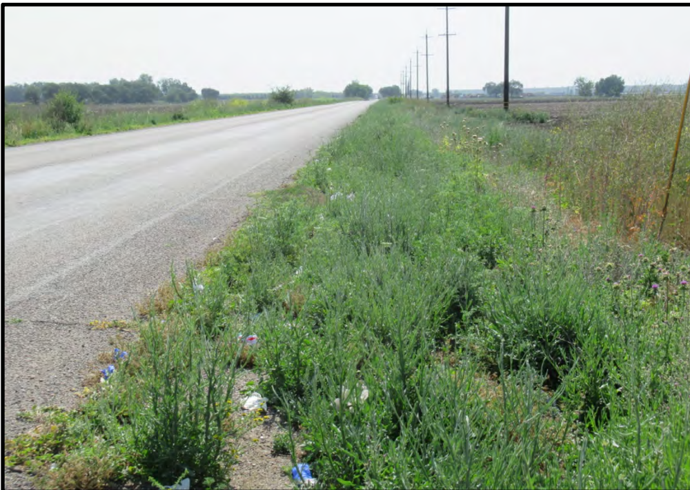
Mariposa Road along the northeast edge of the site, looking southeast; 04/26/22.
