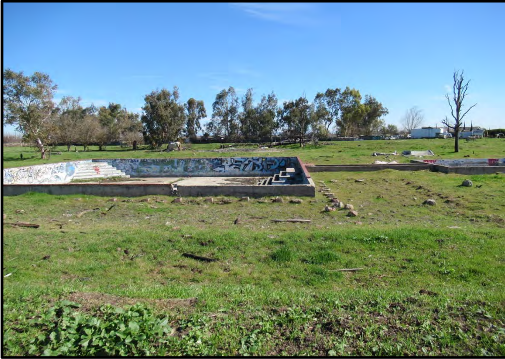
Remnant structure related to a previous aquaculture facility in the south-central part of the site, looking east; 02/22/21.
