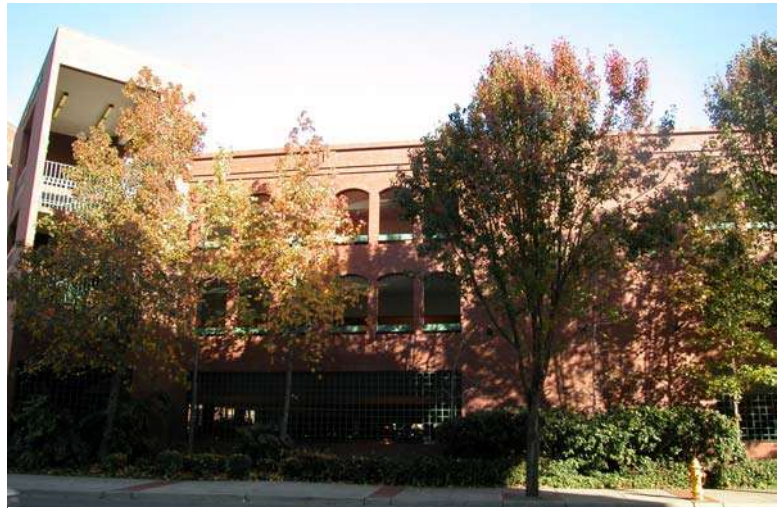
Dense landscaping provides screening for parking structure.
