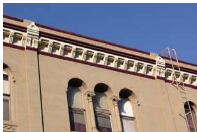
Example of restored cornice detail.
